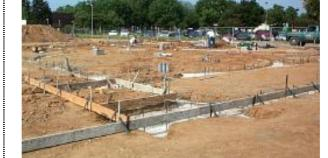
**Curing concrete:** Freshly poured concrete foundations must be left to cure until strong enough to support a newly built structure.
