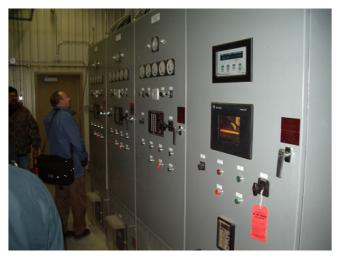
Substation monitoring: To track intermittent faults in an electrical substation, a wood manufacturer logs power levels both pre and postevents
